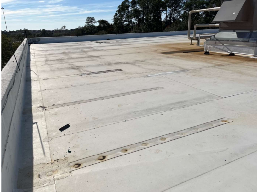
Interseam stripping is installed at the corners to add more fasteners.
